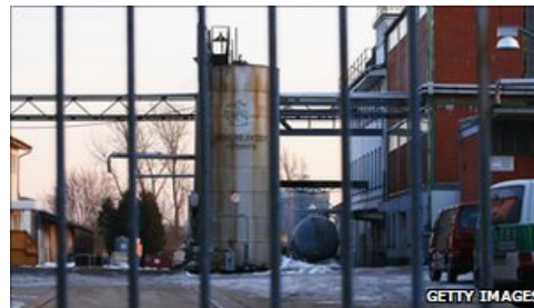
Harles und Jentzsch plant in northern Germany
